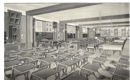
Classrooms in 1897 at the Francis M. Drexel School. Note the gaslights, chalkboards, moveable walls, and the maps and pictures on the walls
